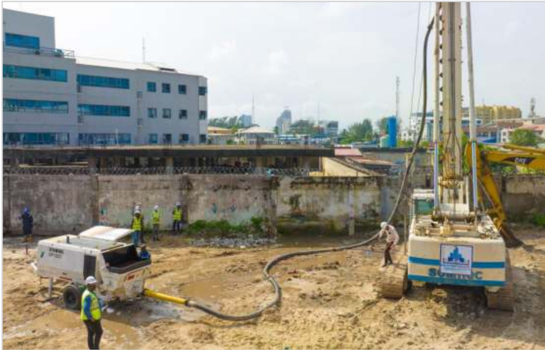
CONTINUOUS FLIGHT AUGER (CFA) PILING RIG
