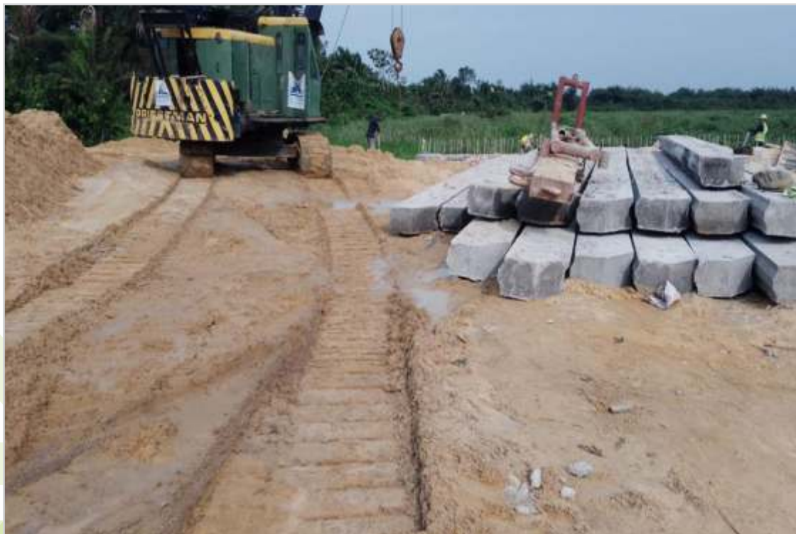
40 TON ROUGH CRAWLER CRANE
